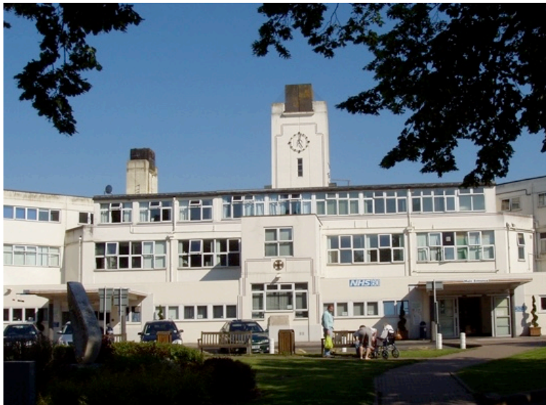
Front view of Kent & Canterbury Hospital
